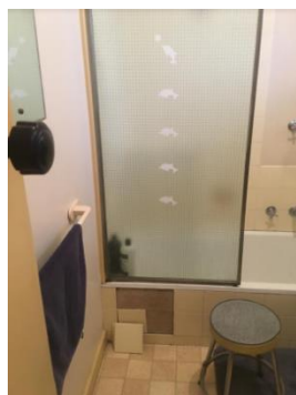
Hole in plaster above bath and tiles falling off in bathroom
